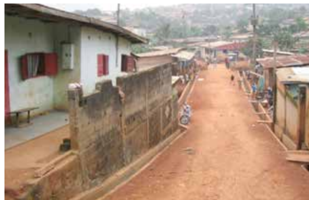
Upgraded road, Yaoundé, Cameroon Photo: © Reinhard Skinner
